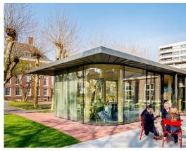
In the courtyard garden next to the Hermitage Museum in Amsterdam a teahouse has opened its doors in April 2014. The new pavilion has a wood structure and a full height glass facade running around the building. Hot bent glass panels at the corners provide an unobstructed view into the urban garden and incorporate the garden into the interior.
