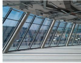
The office building The Curve is a new landmark in the harbor of Amsterdam. The assymetrical stand alone building is transparent and has slanting walls combined with an elliptical floor plan. It contrasts with the surrounding buildings. The form complexity has been the greatest challenge. By efficiently making use of parametric engineering a few details could be designed as principles after they could be applied to many different positions in the building.
