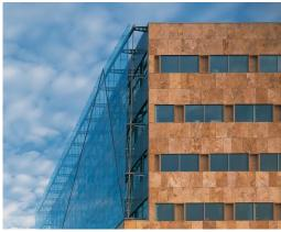
For the headquarters of the Dutch insurance company Zwitserleven in Amstelveen (designed by the Architekten Cie) a second skin facade has been realized and two glass skylights with trusses partly stabilized with innovative glass pressure rods.
