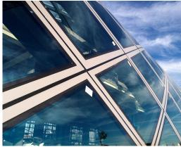
At the Rokin in Amsterdam, Ivy Group has developed two luxury warehouses in collaboration with architectural office Rijnboutt and main contractor Van Wijnen. One of these buildings features a unique rounded roof structure cladded with panels. The structure is 80 meters long and consists of a gridshell with 423 rhombus shaped sandwich panels. The structure houses a restaurant.
