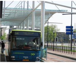
The Delft bus and tram stop roof has been designed using the maximum possibilities of cold warping in vision, resulting in a continuously warped roof which has such a size in length and height to be in harmony with the adjacent shopping centre complex Zuidpoort. The main structure is a tubular steel frame, suspended from 7 conical masts. On the undulating roof plane of round tubular members the glass planes have been fixed and clamped by point supports.
