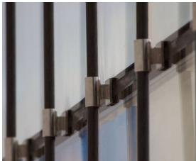
Innovation was the driving force behind the development of the world's thinnest glass facade at the INHolland School of Applied Sciences in Delft. Among the innovative practices are the combination of prestressed aramid cables, hi-tech composite materials, and a load bearing structure inside the cavity of double glass units. This experimental project could be realized due to the exceptional synergy between design and build partners.
