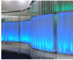
For the Glasstec fair in Düsseldorf Octatube has realized a glass wall for Schott AG, that incorporates several of their new products, such as glass tubes. The undulating wall is 2.8 meters high and 12 meters long. The largest challenge was to realize a transparent wall and maximize the potential of the glass tubes.
