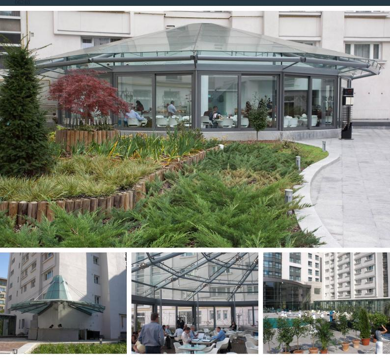
The old hotel Bucuresti, the only hotel in times of communism, has been taken over by Radisson Sas. On the difficult accessible courtyard Octatube has made four glass elements: a subtile glass canopy between the parking garage and the hotel, a glass canopy above a bar, a glass roof on the resaurant and a glass facade between pool and jacuzzi.
