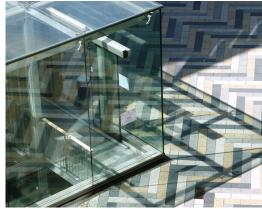
The entrance to the underground bicycle parking garage under the Danzigerkade in Amsterdam is light and transparent. On top of the trusses, stainless steel clamping plates hold the large glass panels in place. The space between the panels is filled so that the glass facades act as a stabiliser. A stainless steel traction cable ensures that the glass panels are held in place. Combined, they form solid construction.
