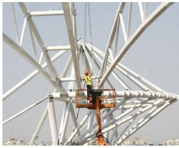
M.Y.S. Architects designed the Cotroceni Park Shopping center, a new multi-story shopping and entertainment complex in Bucharest. The atrium, designed to be the main attraction and spatial focal point of the mall, is an indoor space with a large frame skylight enclosure designed to give full view at a maximum height of 27 meters. Since Romania suffers from frequent earthquakes, the reinforced concrete grid structure was intentionally designed to look majestic.
