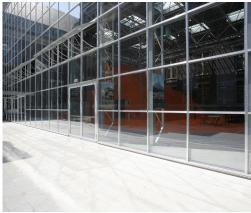
In many applications it is the architect's choice not to use an entirely frameless construction. This has led to Octatube developing lightweight trusses with a (slightly curved) central compression member in the middle and cables above and below. Perpendicular purlins are then provided, delivering the sought-for "floating" effect. Octatube also applies and designs specially formed profiles, such as the steel Stabalux profile, capable of supporting spans up to 3.6 meters with ease.
