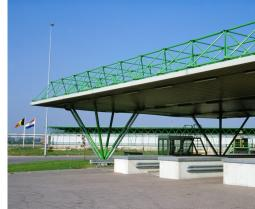
Space frames are lattice structures which work in three dimensions. They are manufactured on an industrial scale. The name Octatube has become linked to the Octatube space frame system. Mick Eekhout invented this system around the time of his finals 1973. Octatube generally produces their space frames in circular steel tubes, but aluminium, solid timber and even cardboard and bamboo have been successfully used on occasion.
