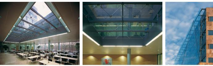
For the headquarters of the Dutch insurance company Zwitserleven in Amstelveen (designed by the Architekten Cie) a second skin facade has been realized and two glass skylights with trusses partly stabilized with innovative glass pressure rods.
