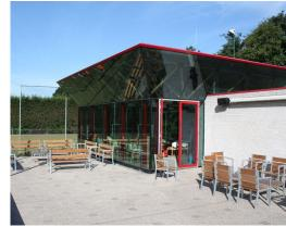
A multifunctional extension for the Hockey & Tennis Club Ring Pass. This extension houses social services like day care. The extension consists of a space frame supported by steel columns. This space frame is made of cardboard tubes and steel balls (Tuballs). It is not the first time Octatube cardboard tubes applied. Octatube developed and produced as early as 2003 space frames with cardboard tubes. This is the first of a permanent nature.
