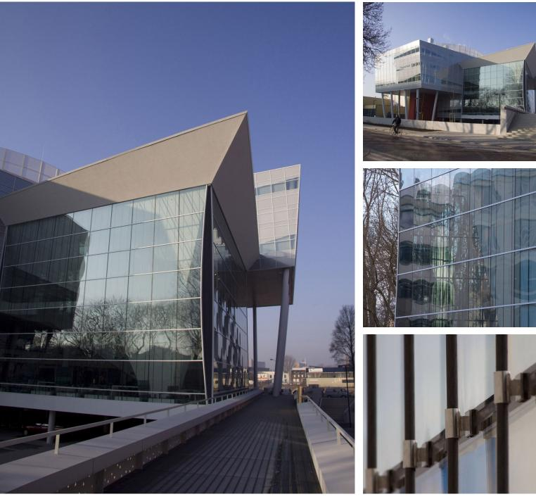
Innovation was the driving force behind the development of the world's thinnest glass facade at the INHolland School of Applied Sciences in Delft. Among the innovative practices are the combination of prestressed aramid cables, hi-tech composite materials, and a load bearing structure inside the cavity of double glass units. This experimental project could be realized due to the exceptional synergy between design and build partners.
