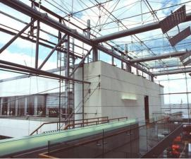
The glass atrium connects an existing office tower with two new office buildings and functions as a central hall for visitors. This glass building part includes a facade, a low atrium roof and two front facades. The weights of the lower roof, stairs and terraces are transferred to the concrete by means of tensile rods in the visible steel structure. The weights of the upper roof and the facade are carried by an integrated truss.
