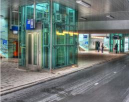
For the renovation of the train station in Alphen aan den Rijn Octatube has constructed several facilities. The glass balustrades that are running along the platform don't have mullions and are fixed at their base. On the platforms of the station three glass elevators are built within a very short timescale because of the proximity of the train tracks. To achieve this, the elevators are designed as prefab elements as much as possible.
