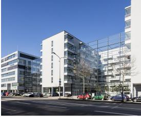
The Studio M2 project, the realization of a large student housing complex, is one of the key projects in a large urban redevelopment. Octatube was involved in the design, engineering, production and installation of three acoustic glass screens that protect the courtyards against traffic noise.
