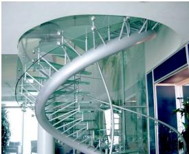
This project consists of a long glass stairs, a glass newel less spiral staircase, glass floors and high glass 'privalite' separation walls. The main load bearing construction of the stairs is a long round tube that winds through the interior of the villa with 6m high halls. This tube is fitted with short tubular jibs on which the laminated glass panels are laid as floorboards.
