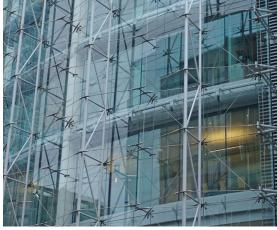
The eye catcher of this eight-storey high building in downtown London is a 25 meter high and 25 meter wide circular structural facade of which the structural elements are visible. This fits the characteristics of High-tech architecture (1990s), where it was fashionable to expose both construction and installations and let them work as architectural and aesthetic element. The high degree of prefabrication is also part of this movement, also known as Structural Expressionism.
