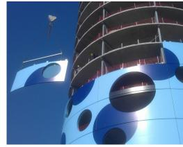
Octatube has been involved in the trajectory of this project from an early stage onwards. By also taking up the engineering and realization of the inner façade, Octatube was able to develop an integrated double façade system. The structural and building physical challenges that were caused by suspending the glass façade on the light weight inner façade were cleared in one swing by replacing the traditional wooden structure with composite GRP elements (Glass Reinforced Plastic).
