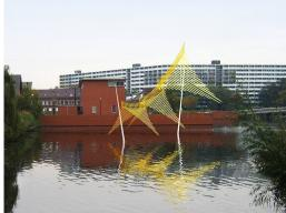
In accordance with the previous design of the Bijlmobiel, one short and one long pylon were set up in the pond. In between the pylons four suspended cables were attached. To these cables overlapping faces were fixed and inter-connected, creating a vivid ensemble of wings. The faces consist of 100 millimeter parallel aluminium strips.
