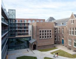
For a student accomodation (designed by KCAP Architects) near the TU Delft, a structurally glazed elevator shaft of 18 meters high has been realised. The steel construction was prefabricated in 3 parts in Octatube's factory which is situated on the University Campus and was transported in these 3 parts to the nearby site. This resulted in a very short installation time.
