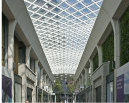
The undulating canopy is 55 metres long and consists of a diamond-shaped grid of steel strips and glass panels. The roof is more than 9 metres above ground level, and also floats a little bit above the adjacent buildings. On Peter Vreedeplein, the roof becomes a large canopy with a more closed appearance of aluminium sheeting and a number of small roof lights.
