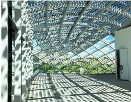
The design for this project is very refined and innovative. The large dome, which is about 45x21x10 meters (lxwxh), consists of two floors and has a free form. Optimizing the shape in 3D and the parametric designing were particularly challenging. Because of the free form of the design, all the parts (steel beams, glass panels, etc.) differ and each time they come together in a different geometric way.
