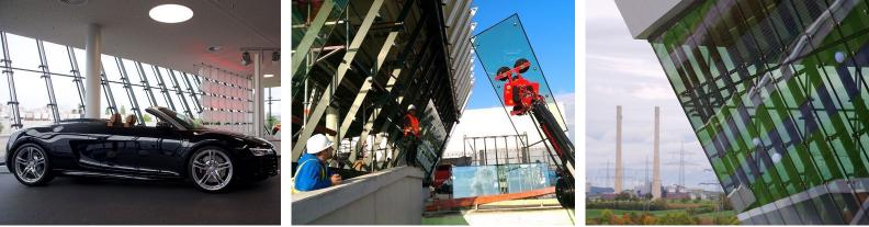
Octatube is responsible for both the steel structure and the glazing: the steel structure consists of very slender strips and the double glass units are point-fixed by means of stainless steel glass nodes. The Audi Sport facility project is characterized by a slanting point-fixed glass façade. The facades are part of the lounge area where the latest models of Quattro GmbH are displayed.
