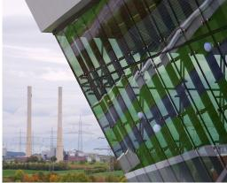
Octatube is responsible for both the steel structure and the glazing: the steel structure consists of very slender strips and the double glass units are point-fixed by means of stainless steel glass nodes. The Audi Sport facility project is characterized by a slanting point-fixed glass façade. The facades are part of the lounge area where the latest models of Quattro GmbH are displayed.
