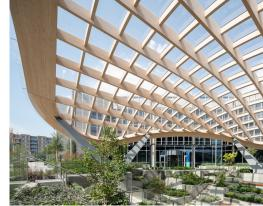
Glulam timber, glass and steel - paired into an elegant and transparent double curved canopy, covers a sunken garden. This one-of-a-kind structure stands on the premises of The Campus, Cherrywood, Dublin. It has a seemingly simple design: three V-shaped columns carry a curved timber grid covered with glass. As the temperature changes, and the wood expands, the glass can move slightly on its profiles. This movement is accommodated in the columns.
