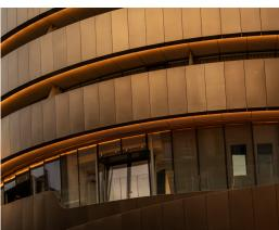
Winding steel ribbons wrap themselves up to form the striking exterior of the W Edinburgh which gives a contemporary twist to the skyline of the historic city. Octatube has realized the stainless steel façade of this striking building. The ribbon is made of Rimex steel: 2 mm thick stainless steel of which the colours and tones vary in different lighting conditions. Due to its curves, the ribbon has a complex geometry with up to 15 cm of torsion in the plating.
