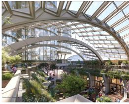
Steel arches and zigzag ladder frames clad with glass panels form the remarkable canopy for the redevelopment of London's 150-year-old Olympia complex. The canopy acts as an above grade level arterial link between the new development plots. It will host bars, cafes and restaurants brining new life to this area of West Kensington. Octatube is commissioned to design and build this eye-catching canopy. The transparent canopy is made of five large steel arches, each with a span of 22 meters.
