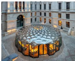
A new and contemporary pavilion has been realised in the Grand Courtyard of The OWO, the former Old War Office in Whitehall, London. Mirror-polished 3D stainless steel panels on the roof give the pavilion its striking appearance. Octatube translated the highly bespoke design of this pavilion into a technical proposal, and was appointed to engineer and built it. The extraordinary geometry of the pavilion has no straight lines and therefor required bespoke solutions and clever craftmanship.
