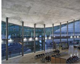
In 2006 Octatube has developed and realized 4000 square meters of exterior glazing, 1500 square meters of interior glazing and 2000 square meters of a canopy for the airport of Valencia. The sculptural terminal has a complex 3-dimensional geometry which also determines the perimeter connections in between the glass and the concrete roof shell. Because of the sunny location sun- and heat-resistant coatings have been applied.
