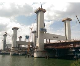
In the context of the A15 highway widening between the Maasvlakte and the Vaanplein, the Dutch directorate for public works and water management realises the largest lift bridge of Europe in the port of Rotterdam. Octatube has realised the fully prefabricated bridge operator house, overlooking the Oude Maas river. It is one of the first projects in which the steel structure is completely executed according to NEN-EN-1090 (execution class 3).
