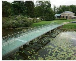
Ruurlo Castle was chosen to be the second location of Museum MORE. Therefore the old wooden access bridge needed replacing. A new high-quality and slim detailed access bridge was designed entirely in glass and bead blasted stainless steel. The contemporary bridge contrasts with the 14th century castle and surrounding park.
