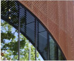
The pavilion with orange-brown corten steel and arches is based on the colour scheme of St. John's Church and the historical facade of the adjoining exclusive shopping mall; Schadow Arkaden. The inner layer of the facade construction is a transparent glass curtain wall façade. The second skin facade consists of perforated corten steel which a sun protection function. Octatube has been hired as a facade specialist because it is a combination of two facades and we were able to realize both them.
