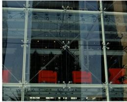
Structural glazed Quattro facade for a showroom in Mexico. The structural steel tubes in de facade have been divided in squares of 2x2 glass panels. A stainless steel "micro-tension" system stablizes the inner glass panels.
