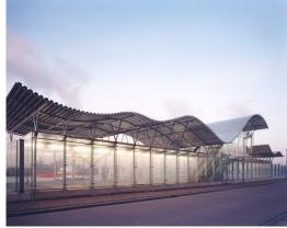
The cruise terminal in IJmuiden is a characteristic building near the sea. Klunder Architect designed a glass volume covered by a hovering and undulating roof. The glass volume consists of elliptical steel portals. The laminated glass panels are fixed by means of Quattro and Duo nodes in stainless steel.
