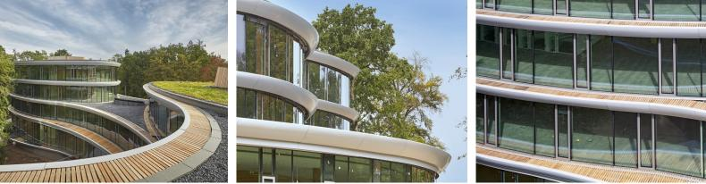
Triodos Bank's new office was designed by RAU Architects and built by J.P. van Eesteren. It is the first large-scale 100% wooden, remountable office building. Three transparent towers run from south to north and are alternately connected on the ground, first and second floors. The composition and shape of the five-storey building is inspired by nature and respects the rhythm of the surrounding flora and fauna.
