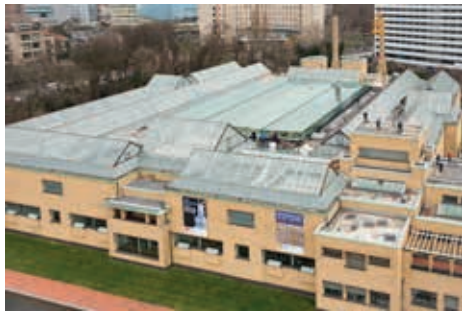
Figure 10: Drone view of atrium roof
